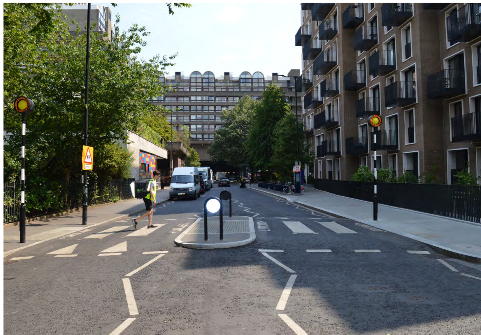
A raised zebra crossing on Golden Lane
